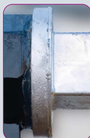
Rotation base of the tower
