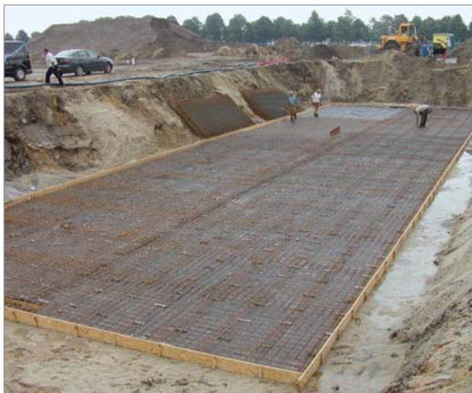
Water collection tank
