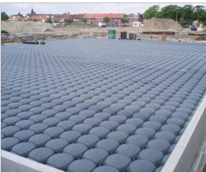
Collection tank under an industrial area
