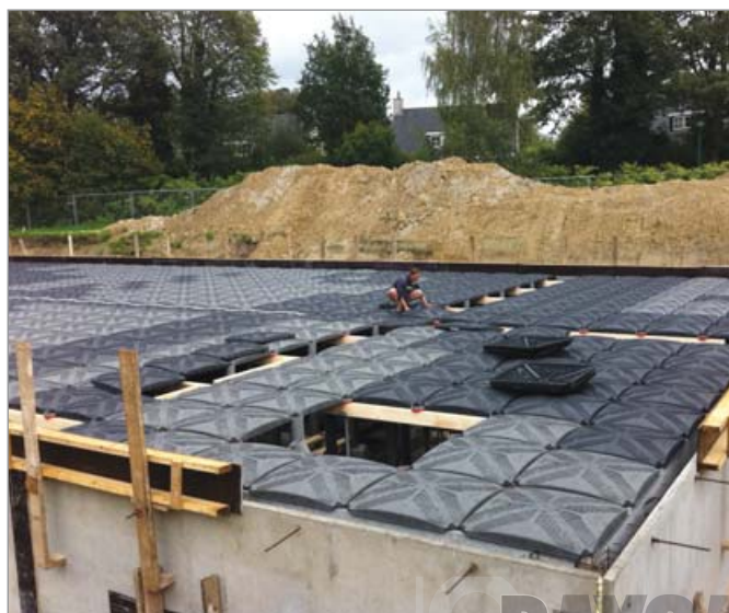
Rainwater collection tank
