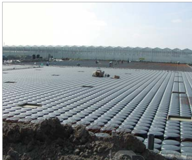
Water collection tank in a greenhouse
