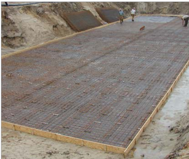
Dispersion tank under a residential area
