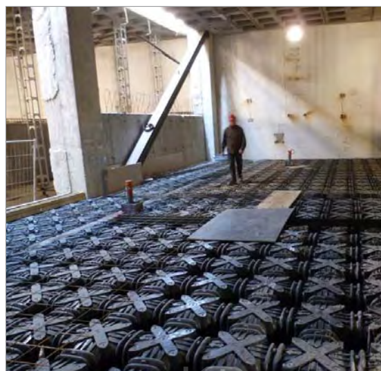
Ventilated interspace for commercial building
