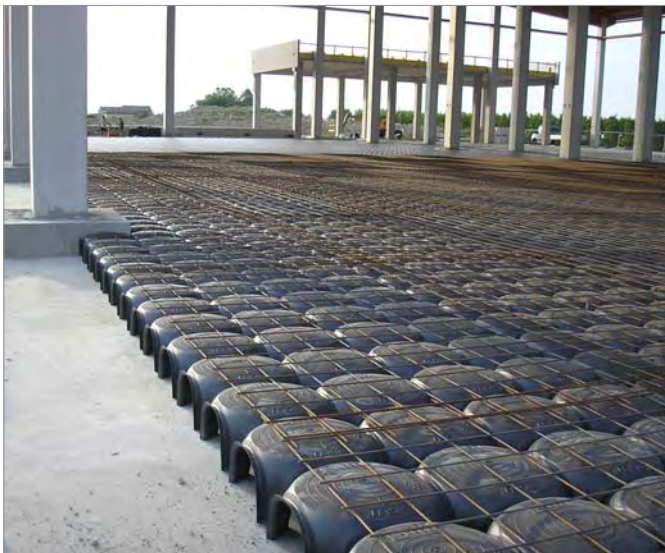
Building for industrial use
