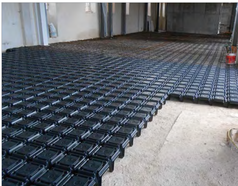
Cascina Triulza restoration - Expo 2015
