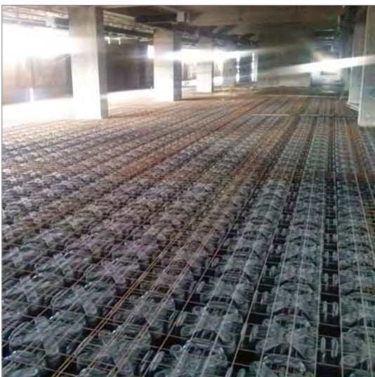
Building for industrial use
