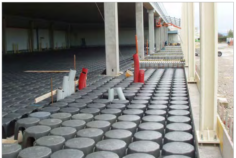
Building for industrial use
