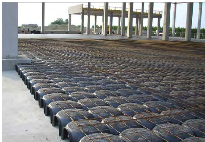
Ventilated cavity for cold room
