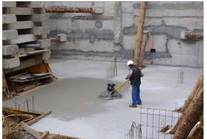
Casting and smoothing
