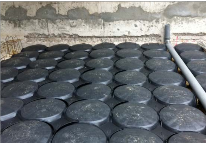
Coffrargile and Beton Up installation
