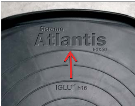
fig. 1 - Dry positioning of the first formwork, the arrow is facing the foundation curb
