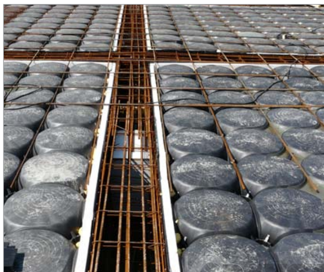
Super raft foundation – system Atlantis in combination with wall formwork
