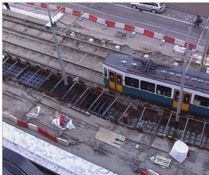
Renovation of a train platform
