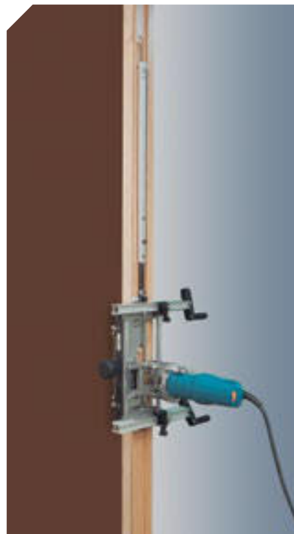
Making the second recess on the frame.
