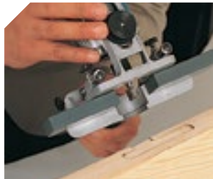
Placing hinges with the ZB93 head.
