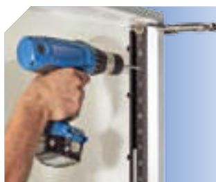
Drilling for placing shelves.
