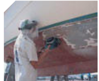
Maintenance work in shipyards.
