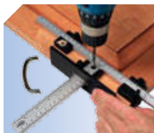
Drilling for door handles.
