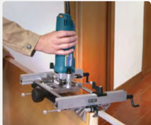
Making the first recess on the door.
