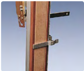
Securing the frames to the template.
