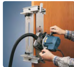
Making side holes for placing the knob, cylinder or other mechanisms.
