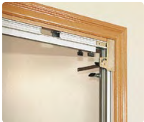
Placing the butt straps using the stops provided.
