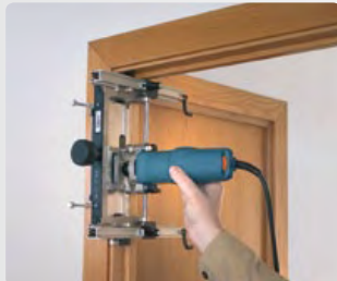
Making the upper recess on the frame.
