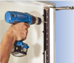
Drilling for placing shelves.
