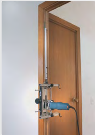
Making the second recess on the frame.
