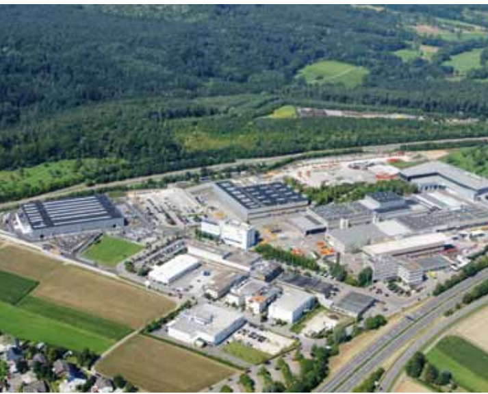
The corporate site of the Putzmeister Group in Aichtal, near Stuttgart
