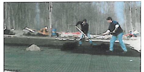
Fig. 5 Relleno con tierra vegetal Filling with soil
