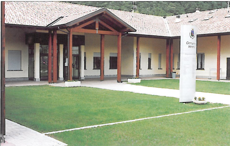
Zonas peatonales y vehiculares terminadas Pedestrian and vehicular zones completed
