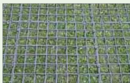
Easy Park just after installation
