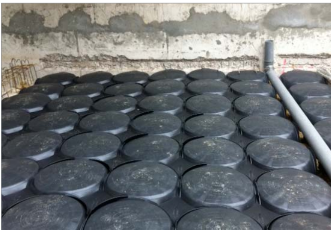
Coffrargile and Beton Up installation
