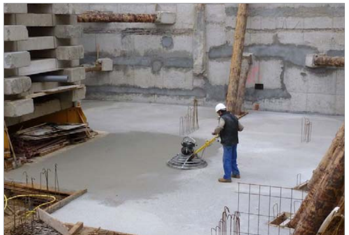
Casting and smoothing
