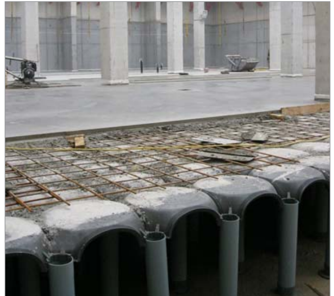
Eni Green Data Center
